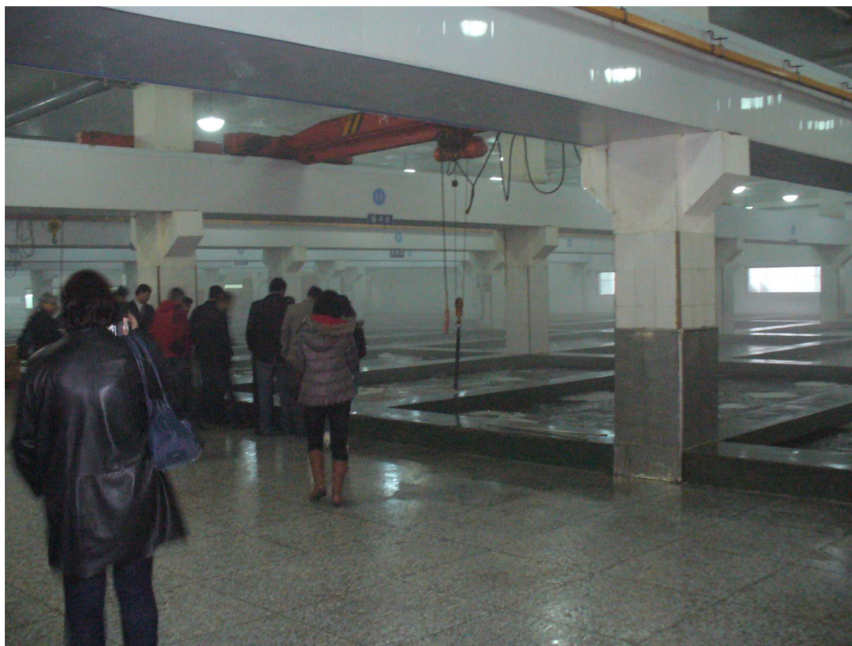
Figure 8: Concrete receiving/holding tanks at the Zhangzidao Fishery group plant.
