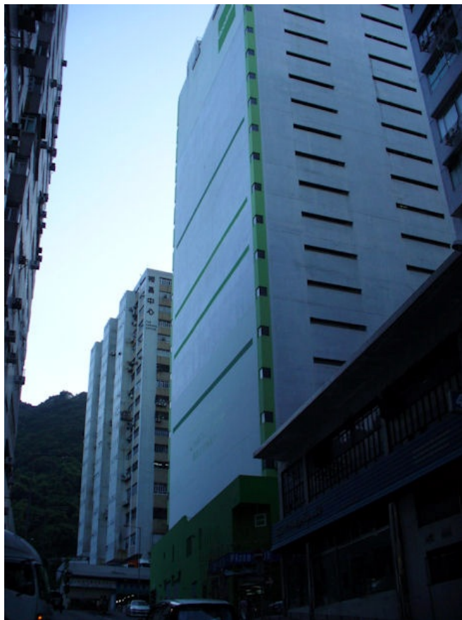
Figure 3: Warehouse where Oceanethix live-hold system is located.
