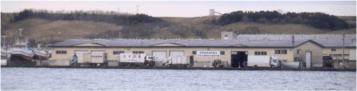
Figure 26: Main unloading jetty backed by the Hanosaki Fisheries Cooperative warehouse and with the winter storage rails to the left.
